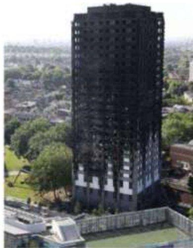
the same tower after the fire still standing
